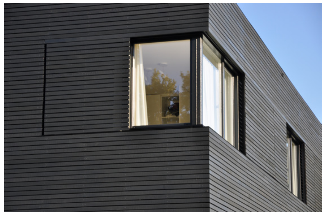
detail northeast facade with slender wooden slats and integrated sliding louvres
